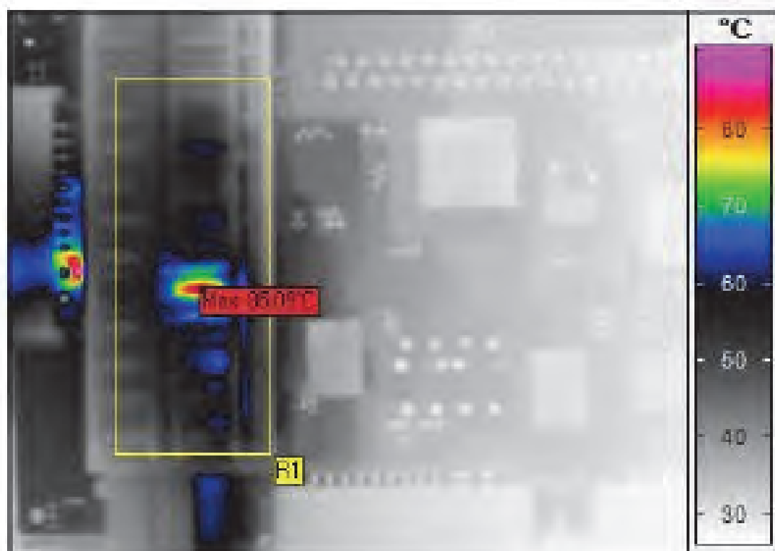
Obr.17 Fuse blok PCB, Mx5
